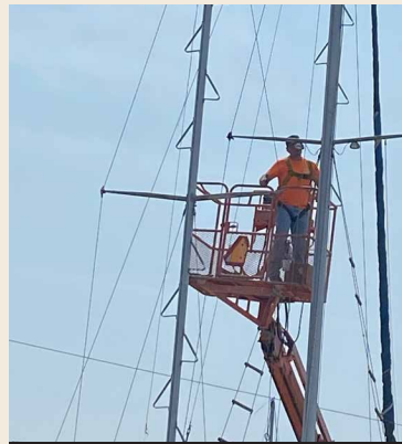
UP IN THE AIR, CHECKING RIGGING
